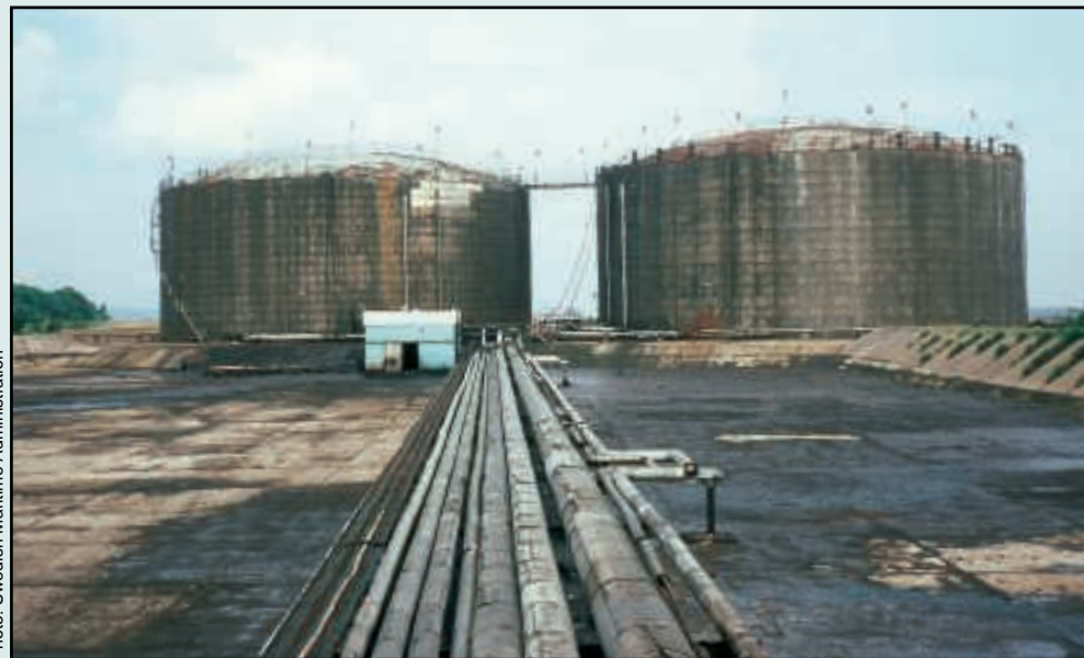
Photo: Swedish Maritime Administration
